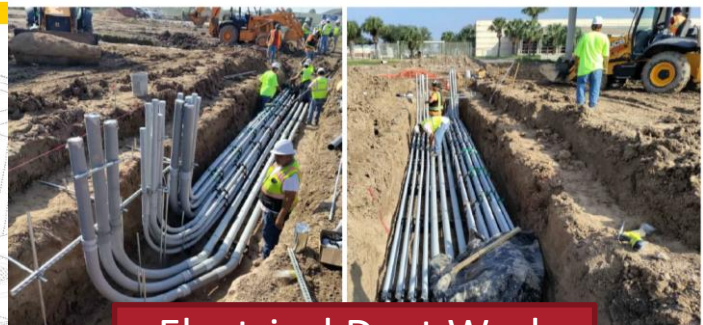
Electrical Duct Work
