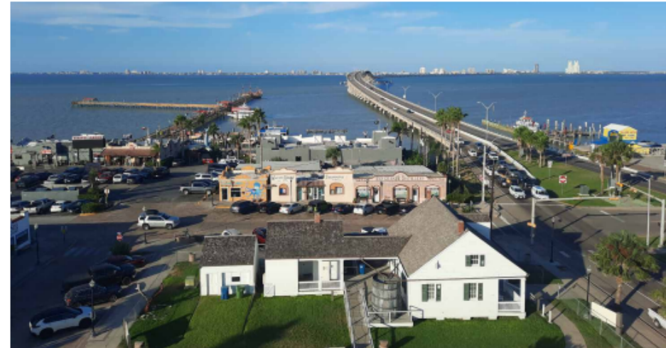
Figure 2. View of Queen Isabella Causeway to South Padre Island
