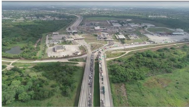
Exhibit 3-33: An aerial of Veterans International Bridge at Los Tomates
