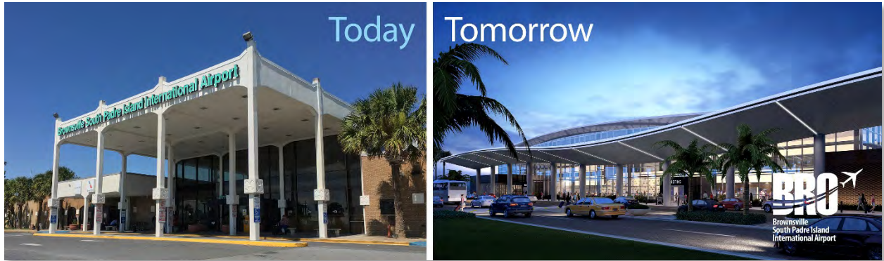
Exhibit 3-37: A before and after comparison of the SPI International Airport after improvements
