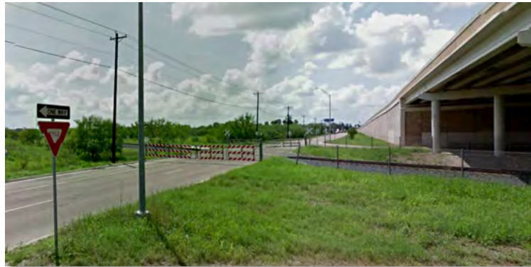
Exhibit 3-27: Barricade at IH 69E/US 77/83 Expressway in Brownsville
