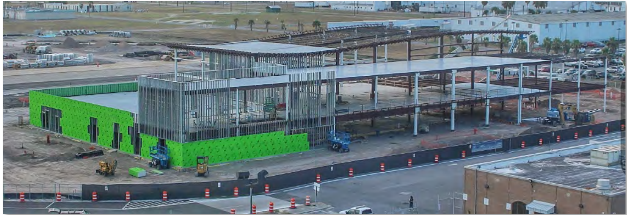
Exhibit 3-40: Construction of the new passenger terminal (August, 2019)
