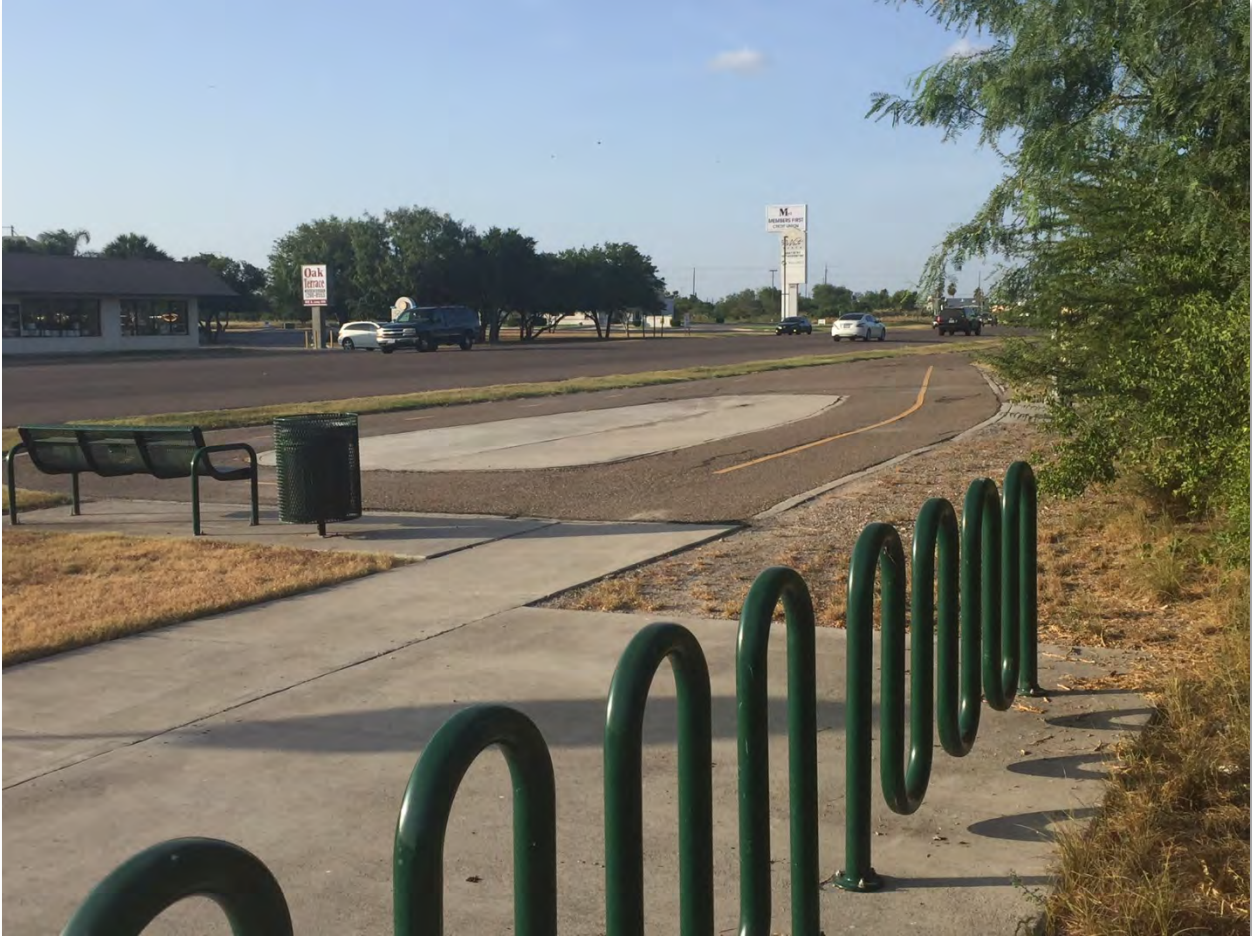
Exhibit 3-24: Protected bike path along Ed Carey Drive, adjacent to Hugh Ramsey Nature Park in Harlingen
