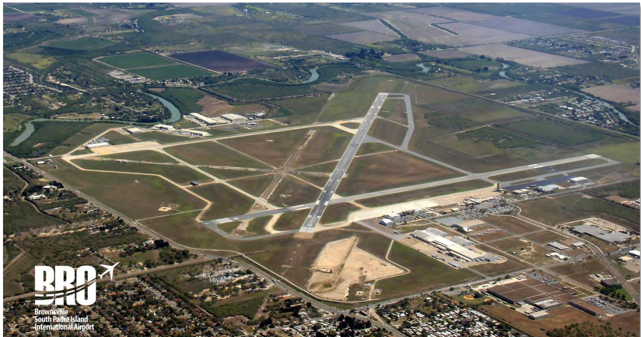
Exhibit 3-38: An aerial of the South Padre International Airport (BRO)
